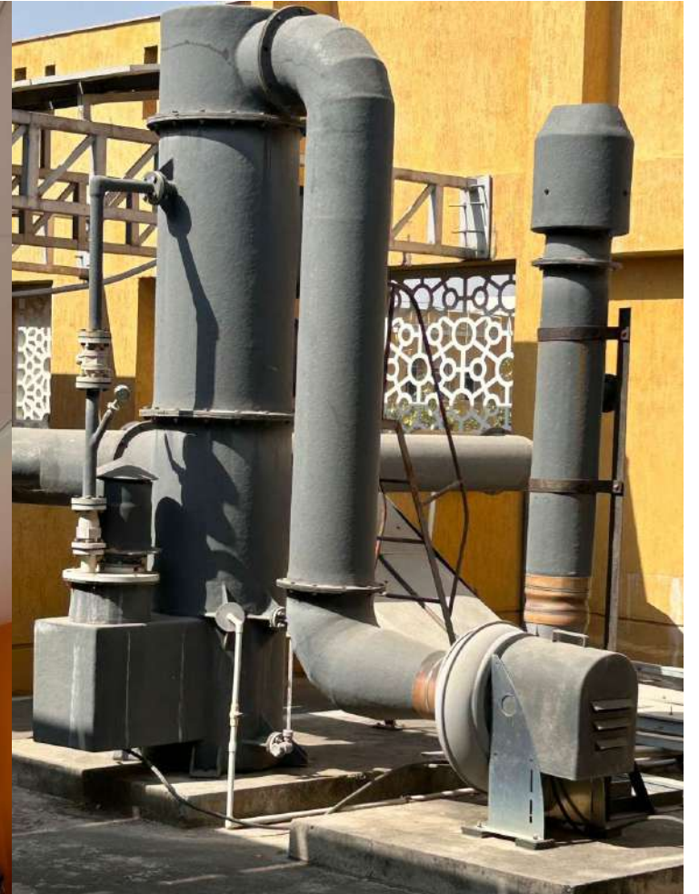
Upgrade HVAC Systems
